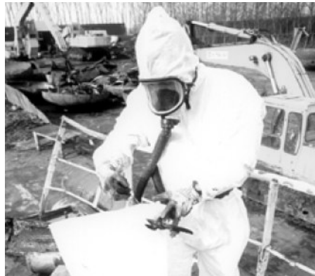
Picture 4: The Netherlands: Asbestos removal from a ship using protective gear. ( www.greenpeace.org )
