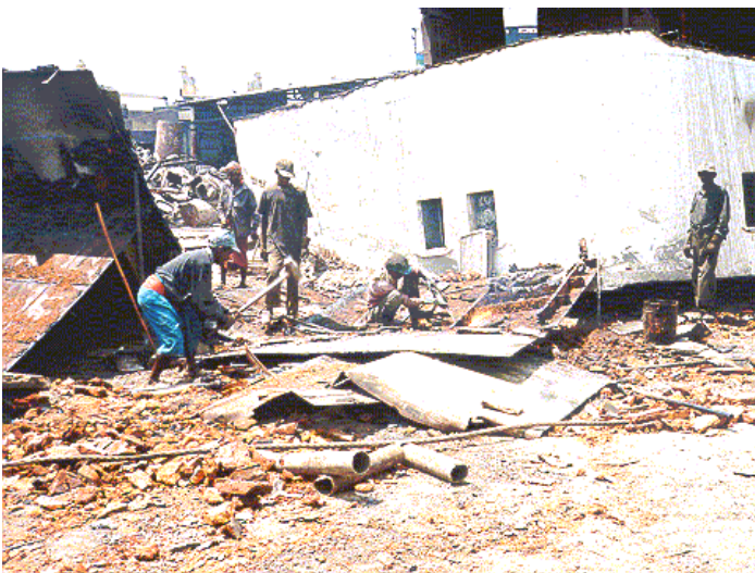
Picture 2: Bangladesh: Ship breaking without protection. ( www.norwatch.no )
