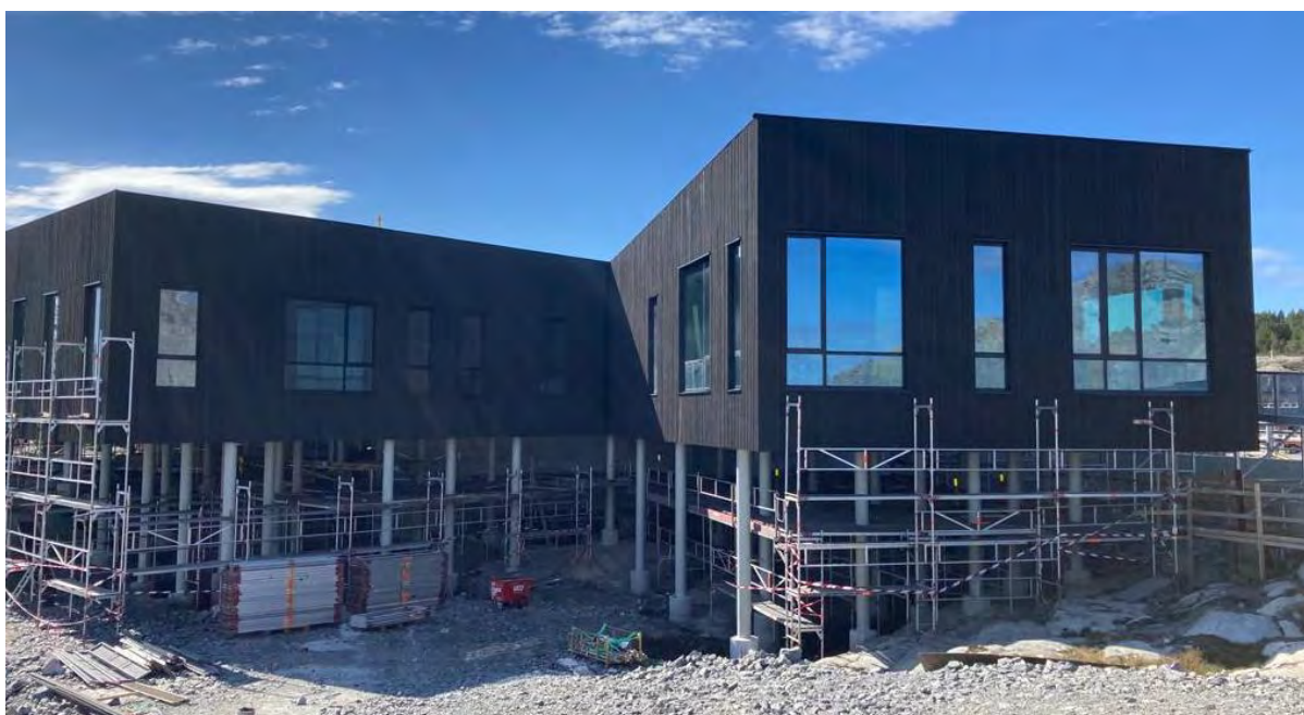
Figure 5.5: Administration building and visiting center, Øygarden
