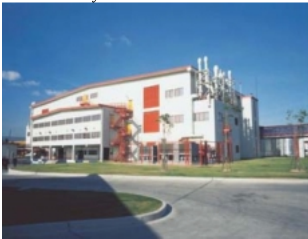
Picture 3 Jotun's new factory
