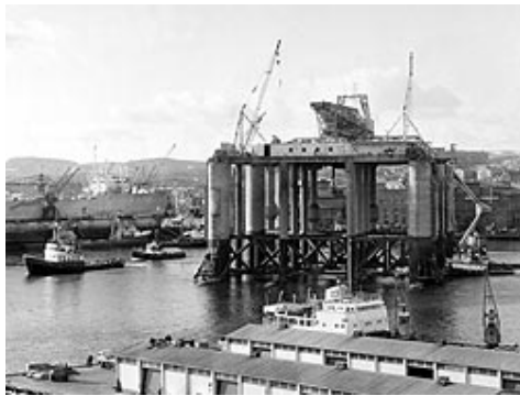
Ocean Viking was built at Akers Mek. in Oslo for exploration in the North Sea.
