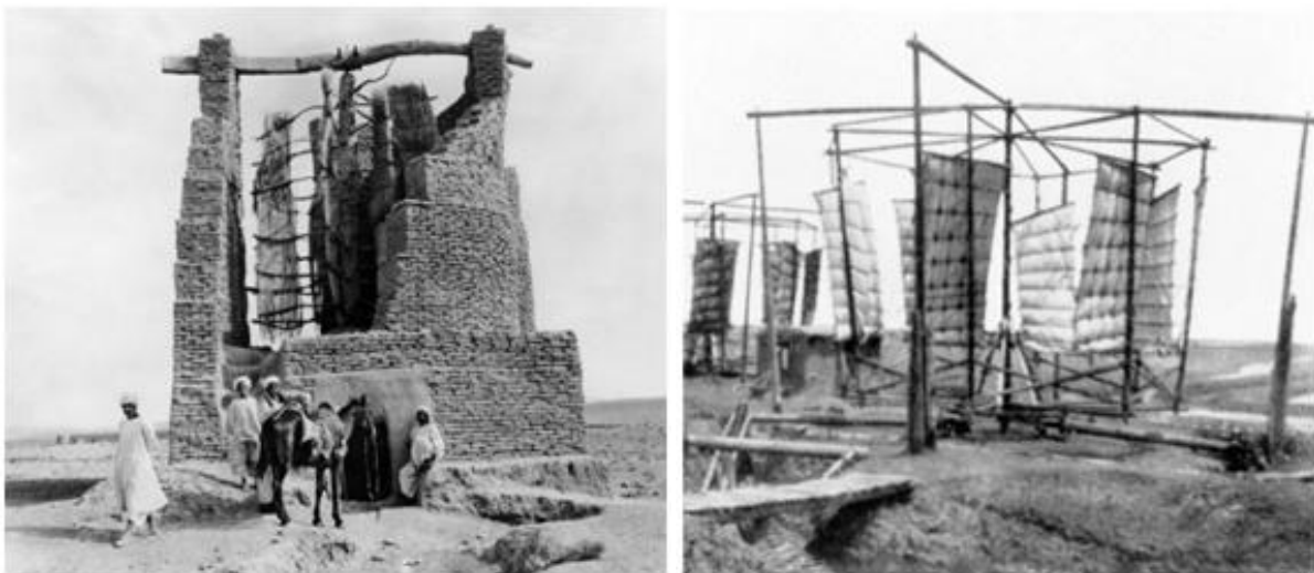
Figure 5 - Wind turbine for grinding grain (left), Wind turbine for pumping water (right) 8
