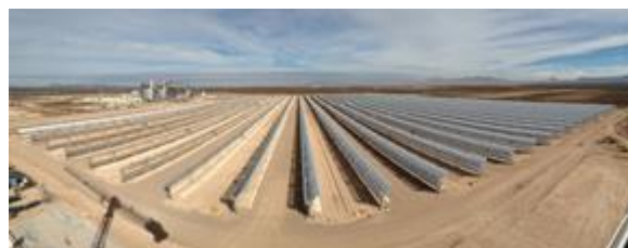
Figure 19: Agua Prieta Hybrid Power Plant (CFE, 2015)
