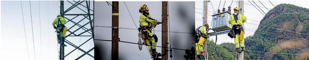
Figure 1. Electricians at work
